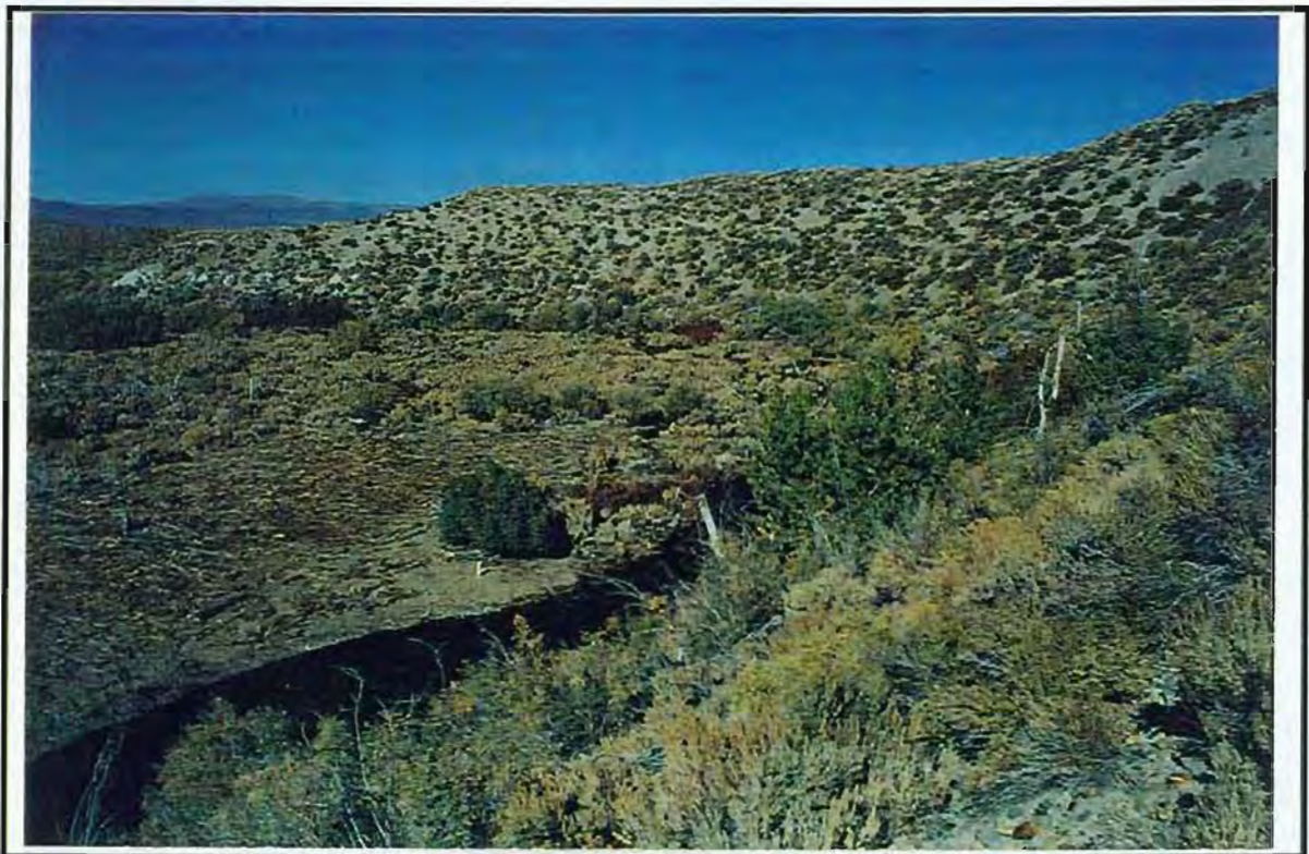
After: The upper section of Channel 10 after the sediment plug was removed and the channel rewatered with ~40 CFS. One of six piezometers is located next to the willow, along the left bank of Channel 10.
