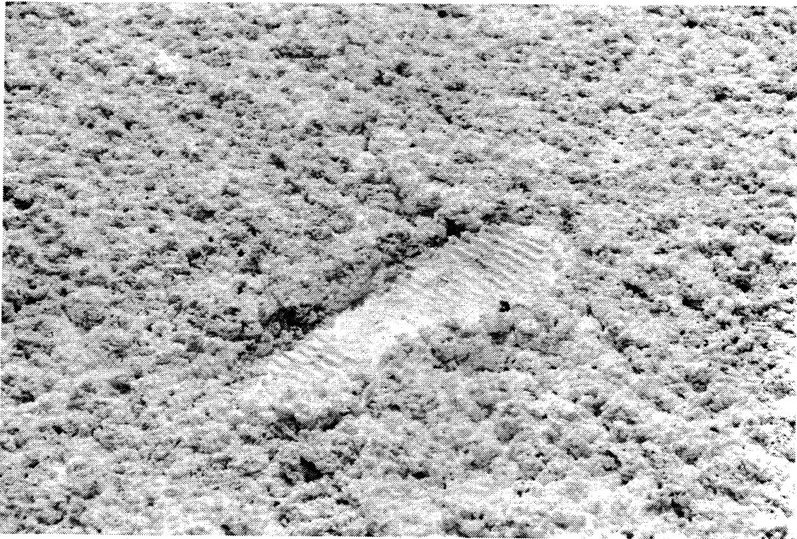
Thick, powdery deposit, lower portion of salt deposits
