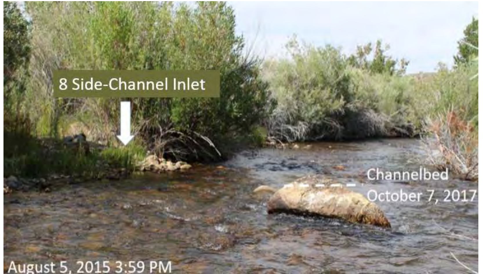
Figure 31. The 8 Side-Channel Inlet on 05August2015 with large boulder and aggraded channelbed elevation surveyed following the RY2017 flood on 07October2017.
