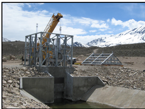
Photo 1: Steel structure assembly
